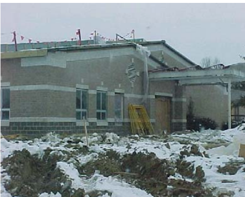
Middle School Addition
