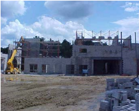
New Jackson City High School under construction
