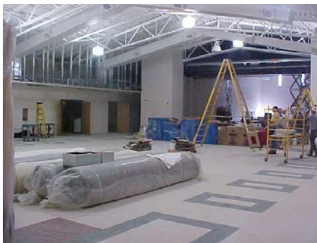
Nearly completed interior at West Elementary
