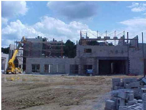
Ongoing construction at Jackson City High School
