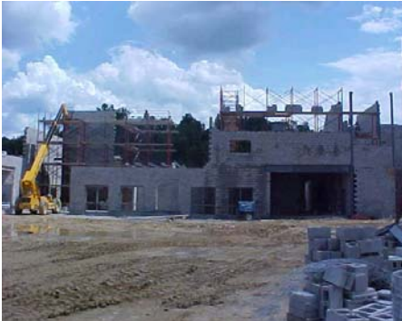
New Jackson City High School under construction
