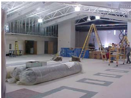
Nearly completed interior at West Elementary
