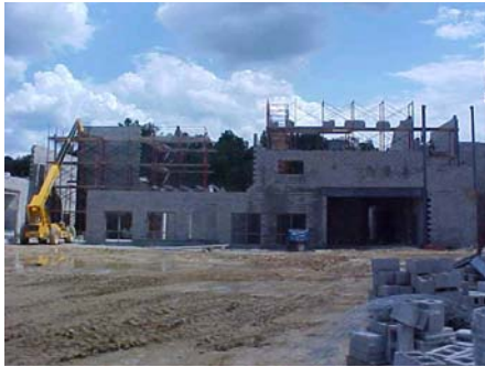
Ongoing construction at Jackson City High School
