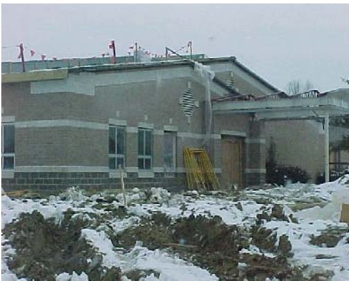
Middle School Addition
