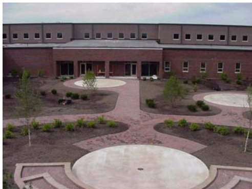
K-12 Facility, Bradford Exempted Village
