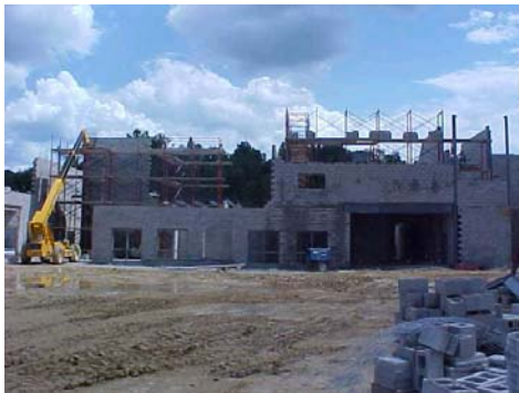
Ongoing construction at Jackson City High School
