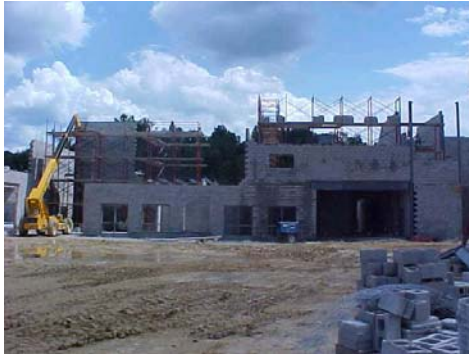
Ongoing construction at Jackson City High School
