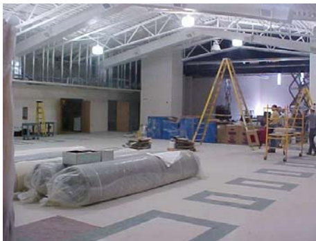
Nearly completed interior at West Elementary
